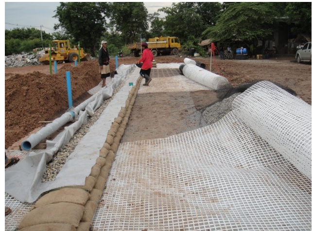
Fig. 5. Construction of reinforced slope involving jute bags as facing.
