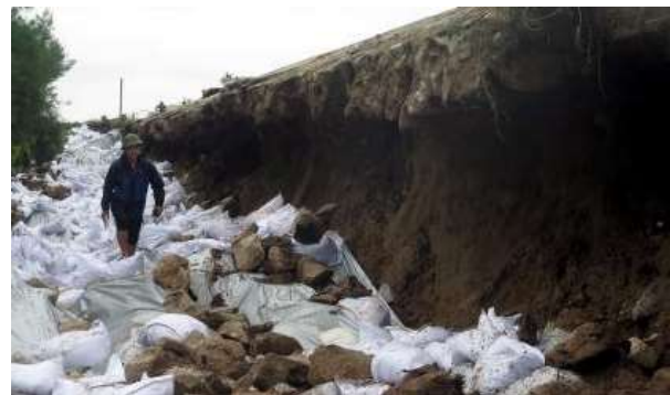
Fig. 1. The broken sea dike in Hai Hau (Thinh Long) by overtopping waves.
