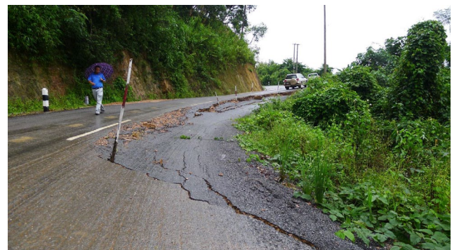
Fig. 3. Pavement failure due to wetting and large volume of water seepage under road pavement at KM 39 to 40 (Case 2).
