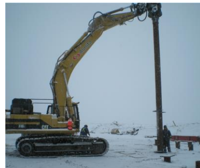
Fig. 1. Installation of the screw pile (Sakr 2010)
