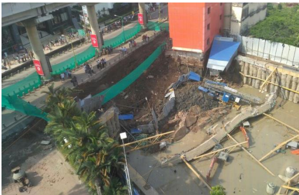
Fig. 1. Failure of Touch Pile System at Kaloor, Cochin
