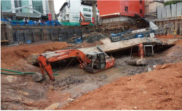
Fig. 2. Refilling of soil after touch pile collapse
