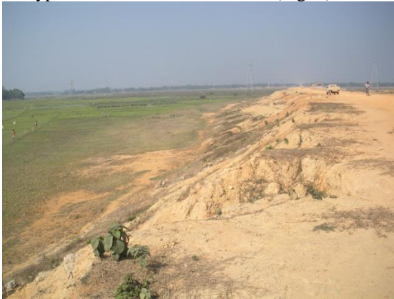
Fig. 3. Heaving of the ground adjacent to the embankment.
