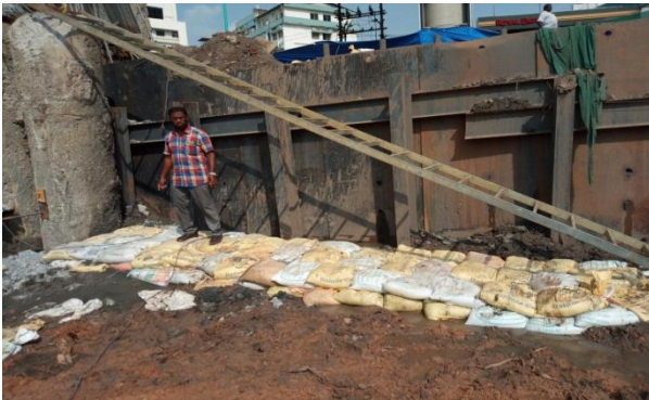
Fig. 3. Two layer sheet pile adopted near public road
