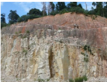
Weathering profile of tropical residual soil (After Lee, et al, 2016)
