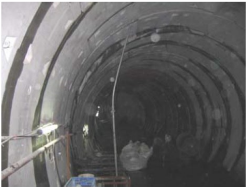
Figure 9 Serious water inflow and dislocation of lining segments inside the up-track tunnel (6:50pm, December 4th, 2005)
