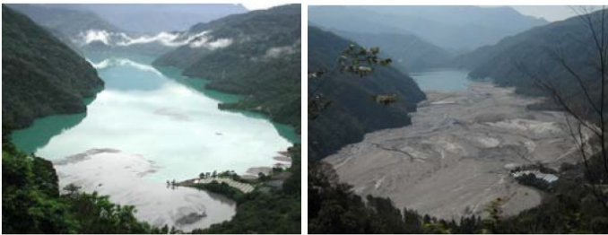
Figure 1 Sedimentation of Typhoon Morakot on Wanda Reservoir in central Taiwan
