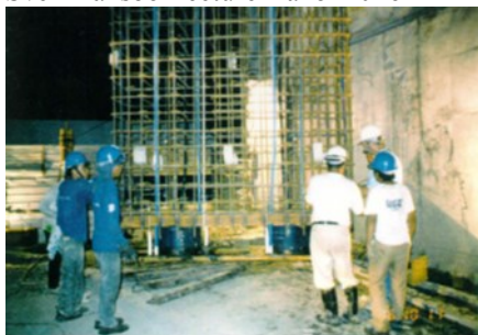
O-Cell Testing : Manila, Philippines
