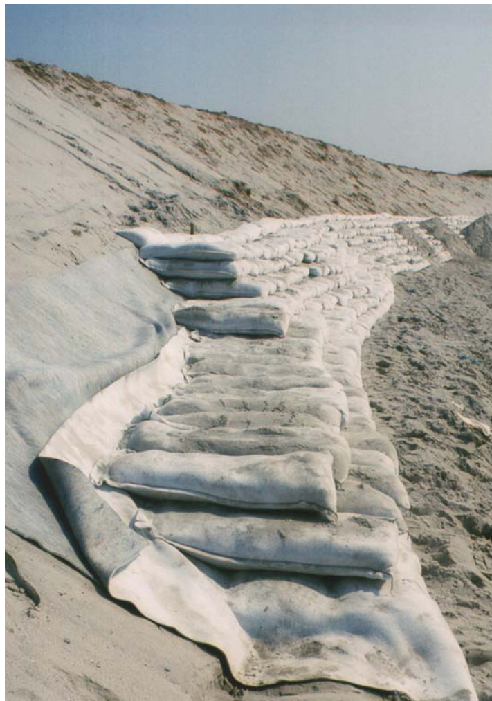
Dune reinforcement in Baltic Sea, (Courtesy Naue GmbH & co. KG)
