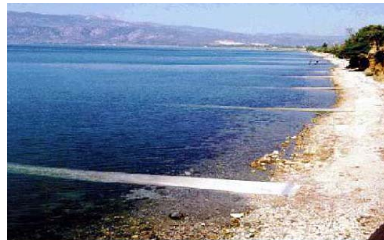
Submerged groins made of geotextile Tubes, Greece
