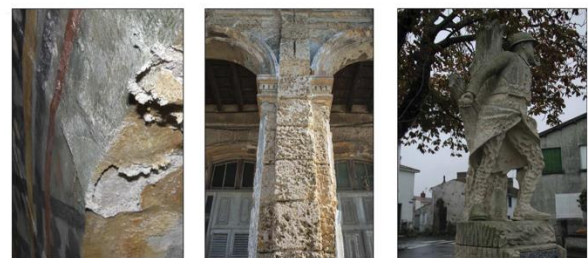
Fig. 4. Examples of salt weathering damages in rocks. Modified from Platt et al. (2004).
