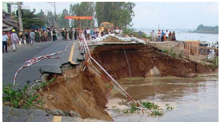
Example of erosional scene of river bank in the Mekong Delta
