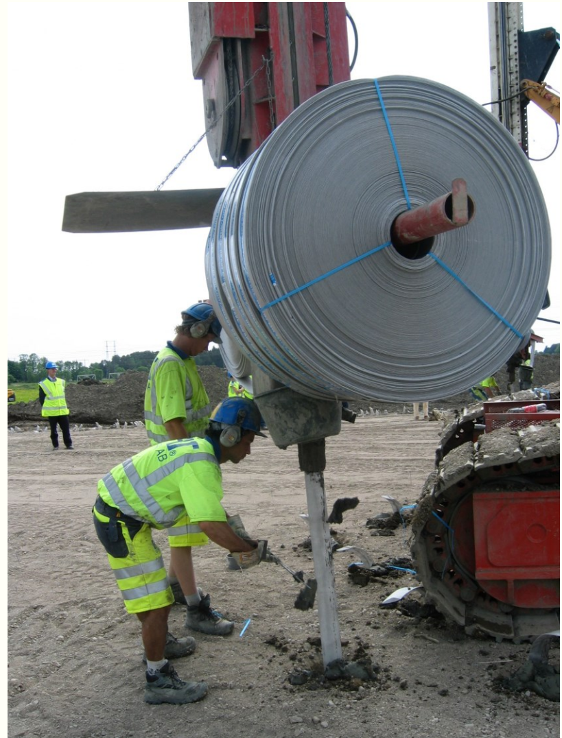
Drain Installation in Uppsala, Sweden
