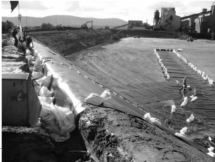
Lined Tailings Dam - Construction
