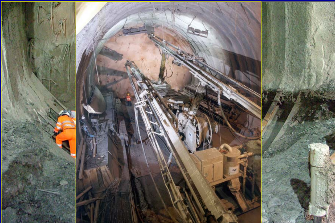
Full face excavation method
