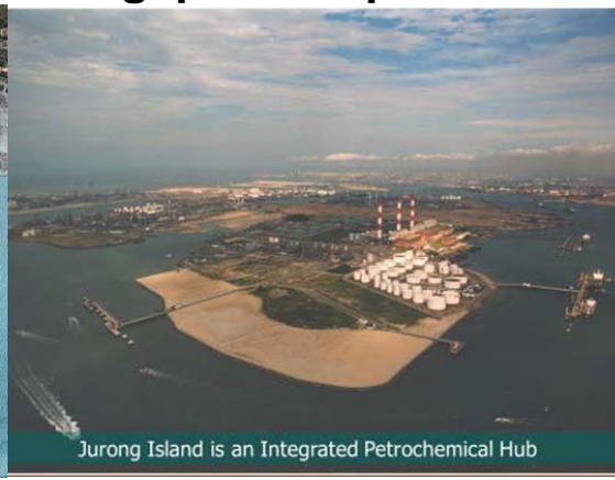
Jurong Island formed from merging 7 islands; ground improvement mostly vibro and stone columns with dynamic techniques
