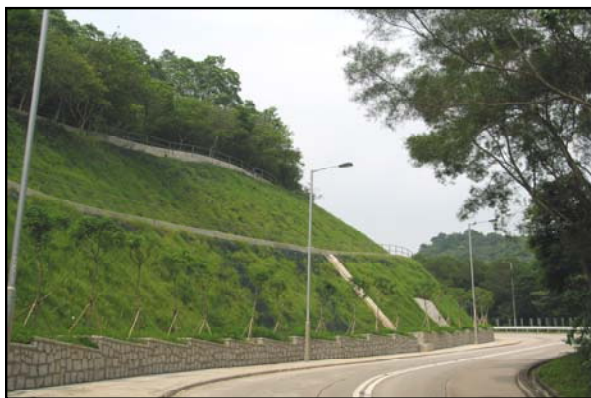
Figure 25 – A slope with landscaped treatment implemented during upgrading
