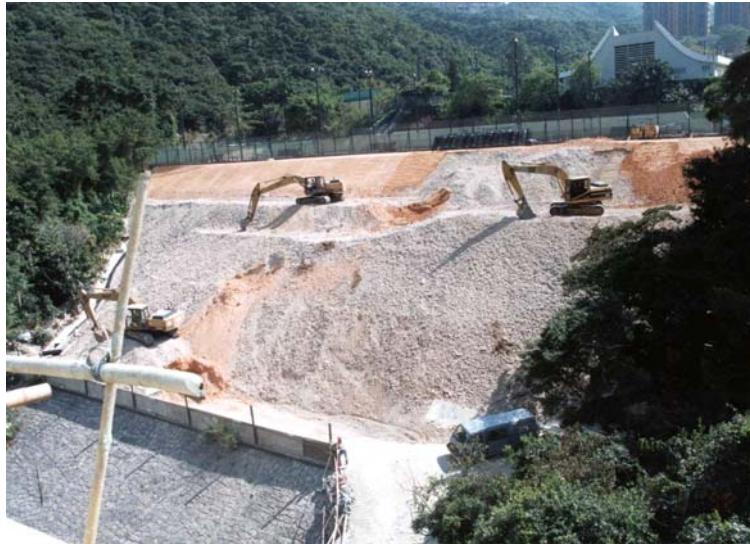
Figure 11 – Recompaction of granular fill in upgrading a loose fill slope
