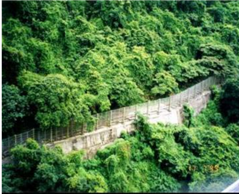
Figure 17 – Boulder fence at Mid-levels
