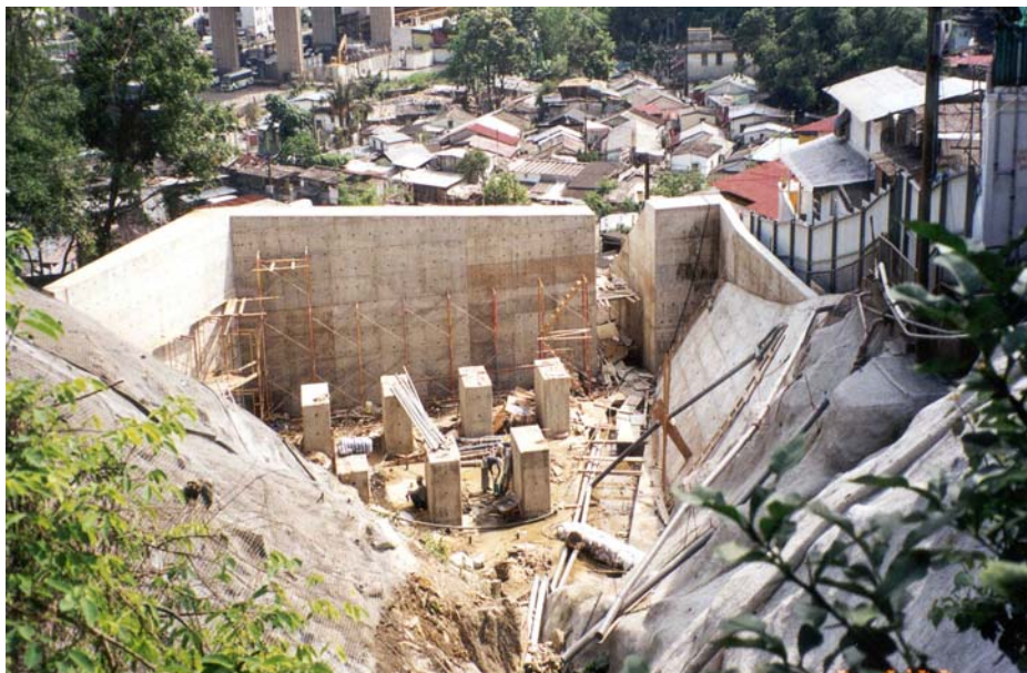
Figure 16 – Check dam built in Sham Tseng San Tsuen
