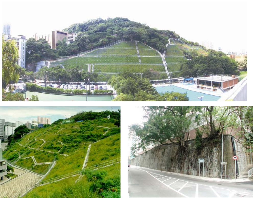
Figure 10 – Examples of vegetated slopes and an upgraded masonry wall with wall trees preserved
