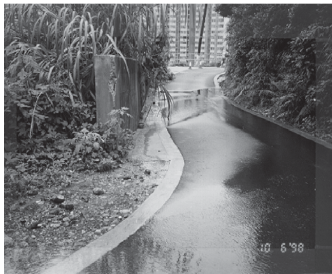
Figure 7. Ponding due to poor surface drainage provision
