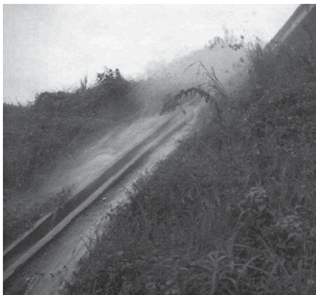
Figure 6. Over-spilling due to inadequate surface drainage detailing
