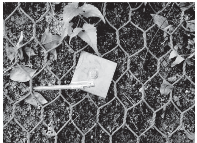
Figure 7. Details of the use of steel wire meshes in conjunction with non-degradable erosion control mats
