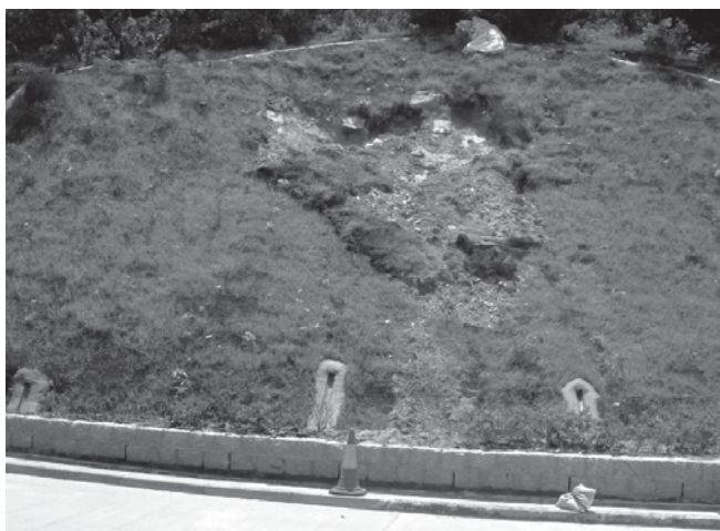
Figure 29. Shallow failure at a completed soil-nailed slope
