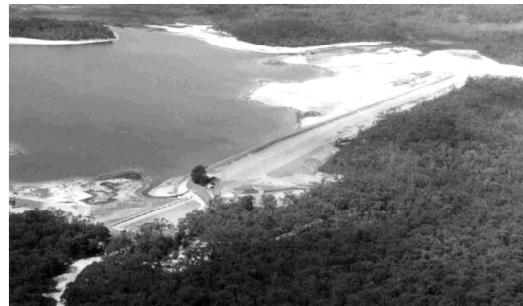
AERIAL VIEW OF THE COMPLETED WARTOOK EMBANKMENT REHABILITATION Primary spillway and new outlet works in the foreground
