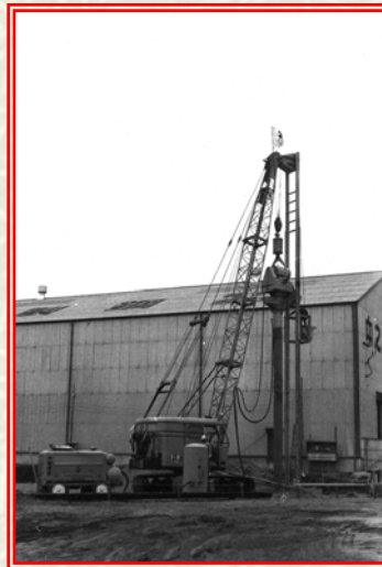
SCP machine with vibrating compaction technique in 1959.
