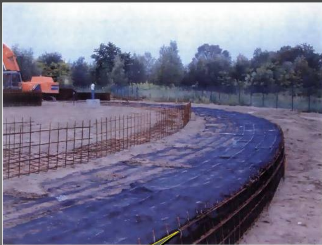
Reinforced earth wall
