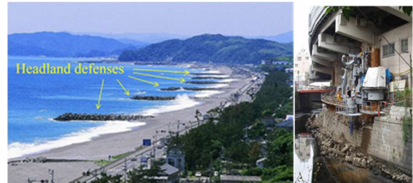
Application of Press-in Method to Coastal Levees in Kochi Coast as Countermeasures against Liquefaction, after Y. Ishihara et. al, 2020.
