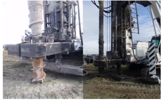
Figure 10 Omega pile installation, test pile instrumented on the reinforcement cage at 6 depth locations.
