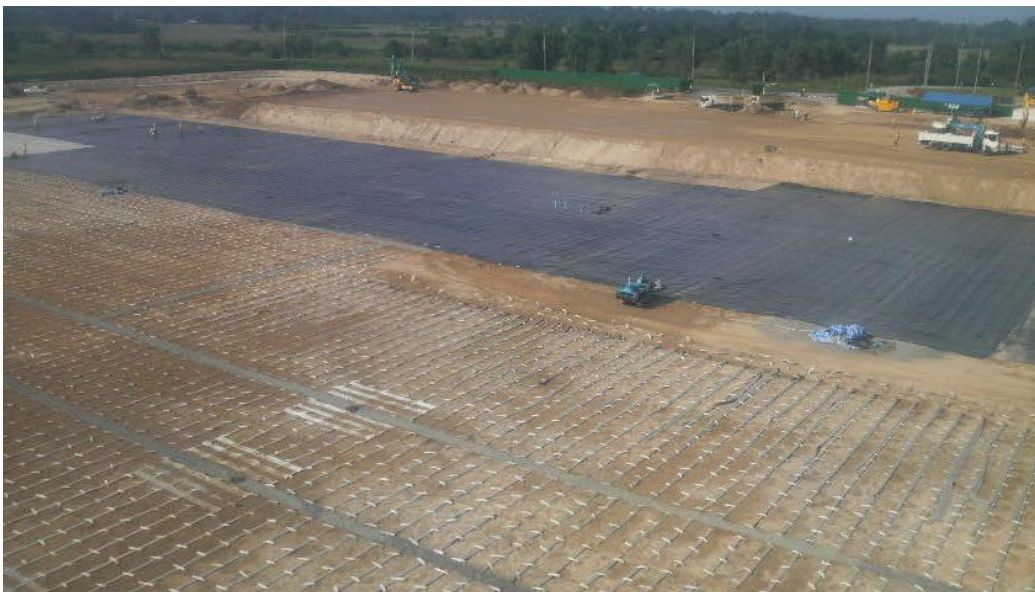
Vacuum consolidation with air-water separation system in Nakhon Si Thammarat Province
