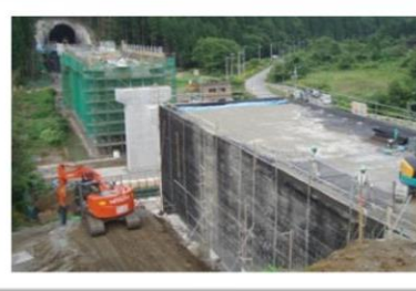
Fig.3: Geosynthetic Reinforced Soil Structure (GRS) in High Speed Rail After Tatsuoka et al, 2014)
