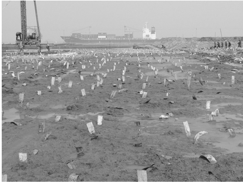
Install a layer of sand blanket and vertical drains
