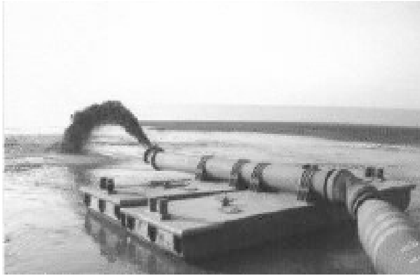
Land reclamation using dredged clay slurry
