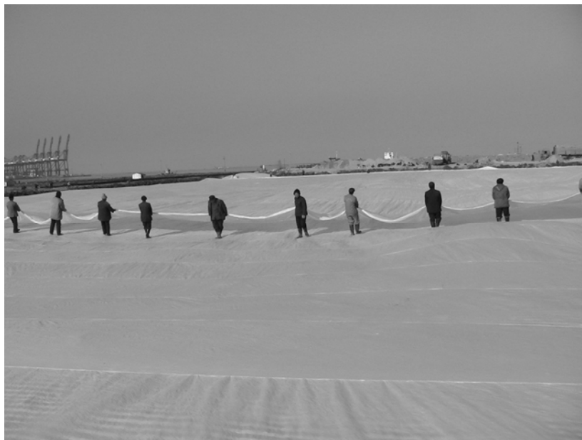
Installation of 2-3 layers of membrane
