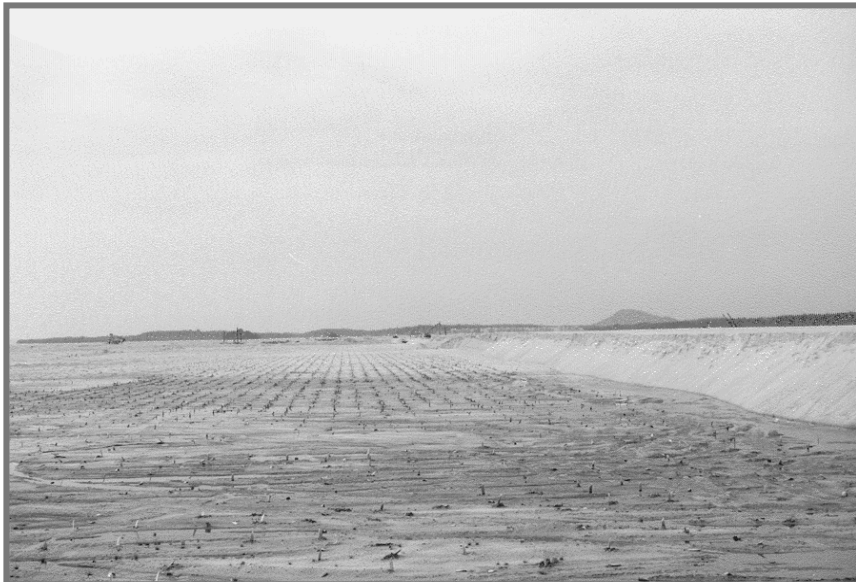
Area Installed with Vertical Drains
