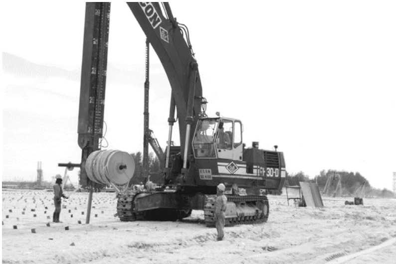
Installation of Vertical Drains
