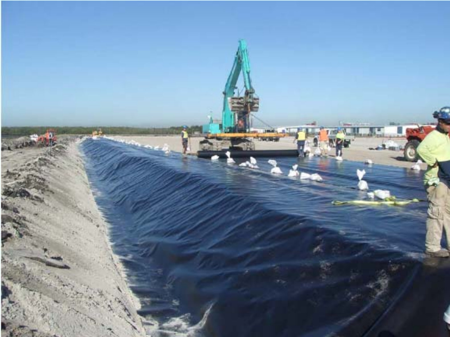
HDPE membrane installation
