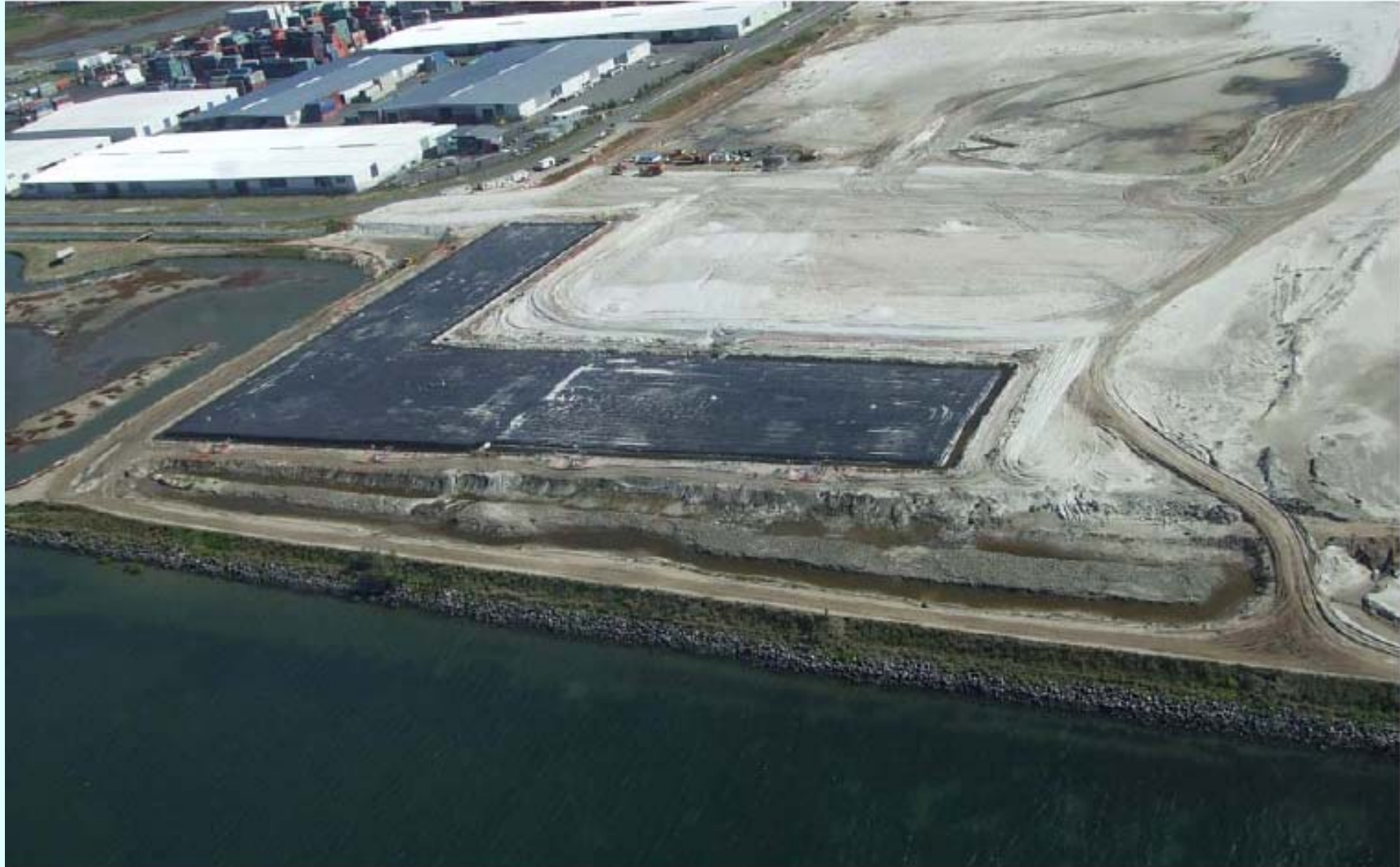
Austress Menard trial sections
