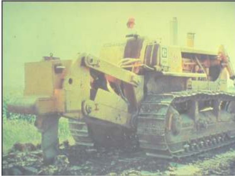
Pavement Ripping with Dozer
