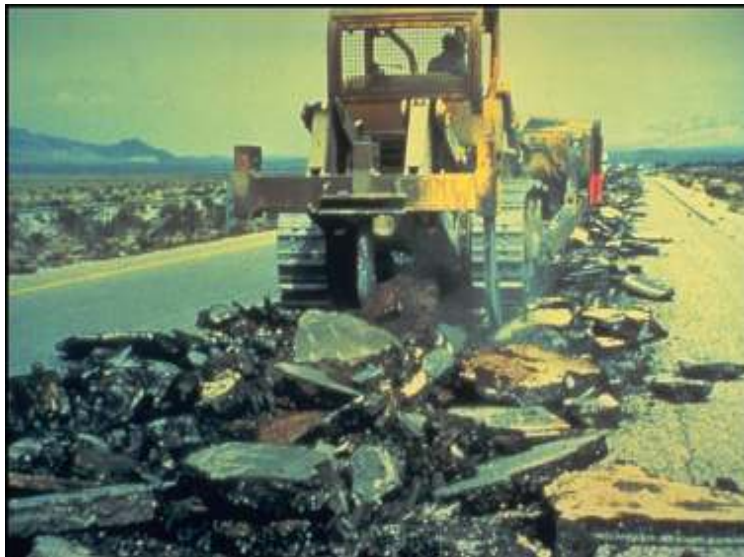
Dozer with Rear Mounted Ripper Tooth
