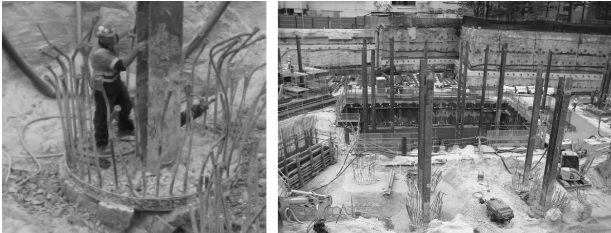
Figure 11: Plunged columns and tower piles after bulk excavation
