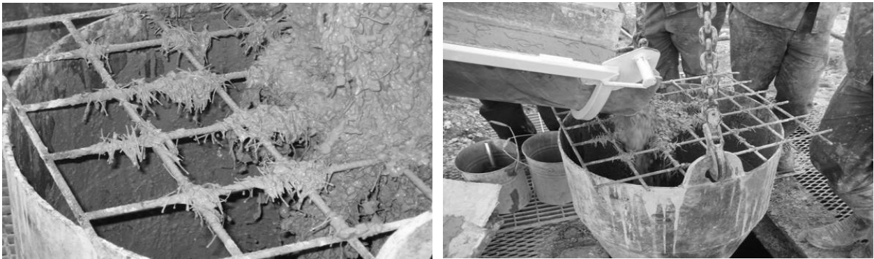
Figure 8: Synthetic fibers added into the concrete mix increased the tensile strength but reduced the concrete workability.
