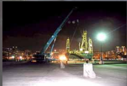
Lifting a jack-up barge across the bridge over Kai Tak Nullah
