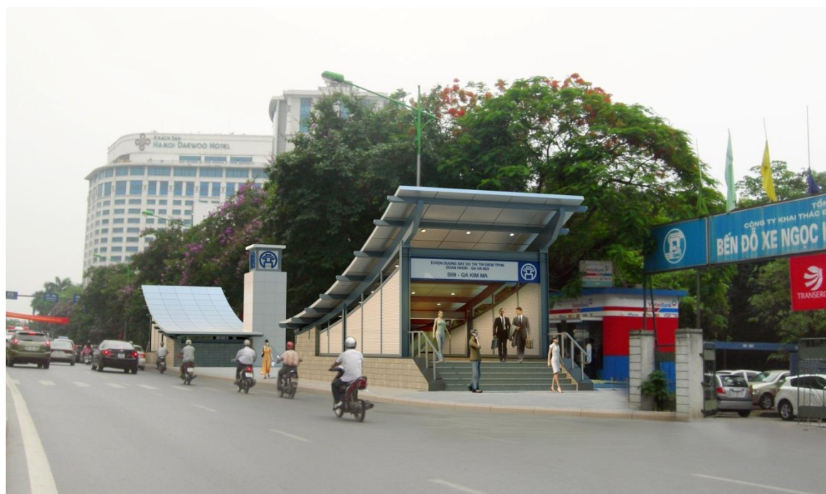
Typical Station entrance
