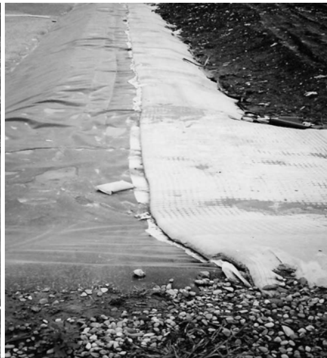
Concrete Filled Geotextile Mattress Protection Layer
