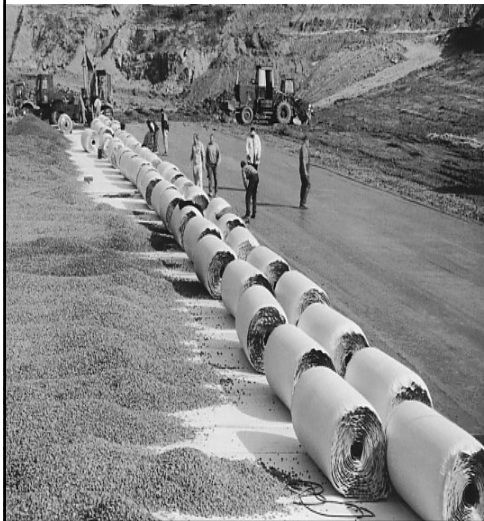
Sand Filled Geotextile Mattress Protection Layer
