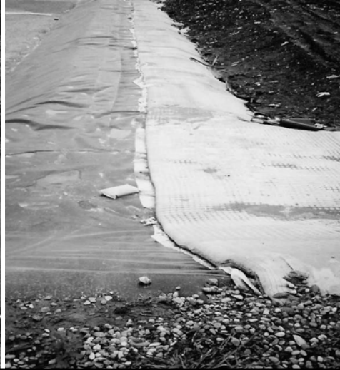
Concrete Filled Geotextile Mattress Protection Layer
