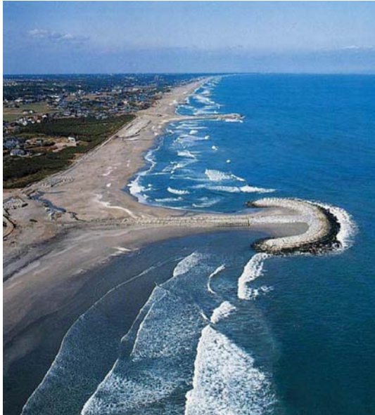
Figure 5 Headland type concrete structures to protect coastal dykes and maintain sand beaches from erosion in Ibaraki, Japan
