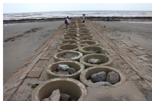
(d) Placement of cellular type of concrete with crushed stones
