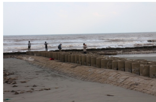
(c) Placement of cellular type of concrete
