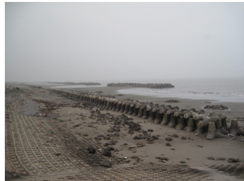
(a) Typical placement of concrete armor blocks
