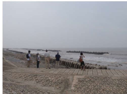
(b) Multiple placement of concrete armor blocks
