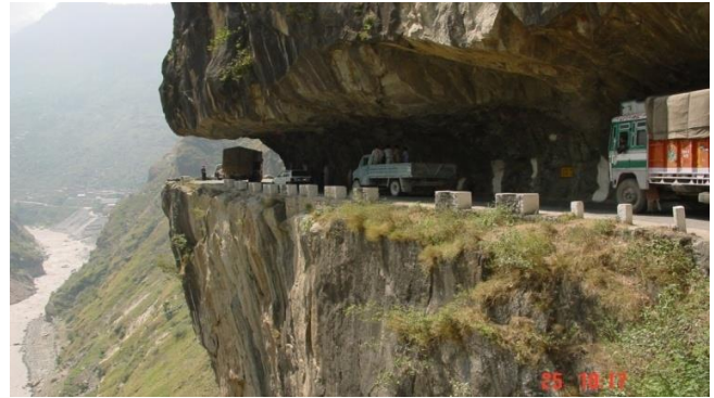
Figure 8 Road construction on rocky mountain in Himachal Pradesh, India remain undisturbed till stability of the rocks are tested by earthquakes and other hazards in the vicinity
