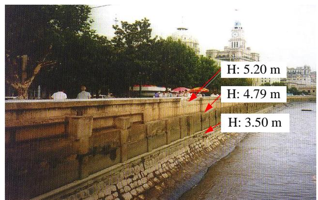
Figure 12 Photo of floodwall along Suzhou River
