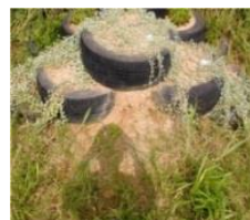
Filling: Soils Placement: Three layers (stepped)
