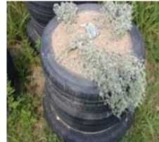
Filling: Soils Placement: Three layers (vertical)
