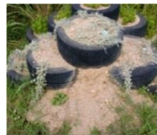
Filling: Soils Placement: Three layers (stepped)
