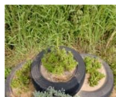
Filling: Soils Placement: Three layers (stepped)
