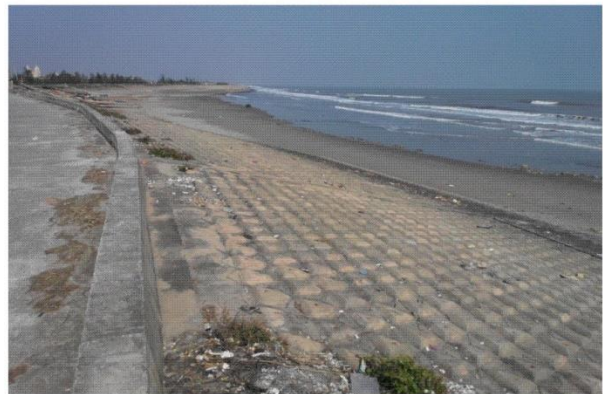
d) Concrete revetment
