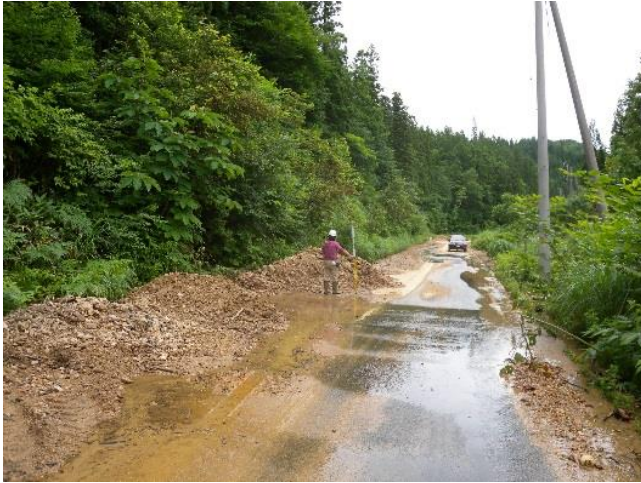
Photo 3 Sediments transported by slope failure
