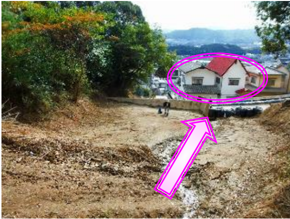
Photo 4 Relation between mountain stream outlet and residences in debris flow in Hiroshima
