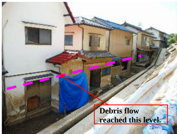
Photo 5 Damaged residences in debris flow in Hiroshima
