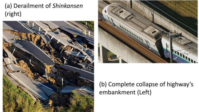
Photo 1 Damage to a railway and a highway
