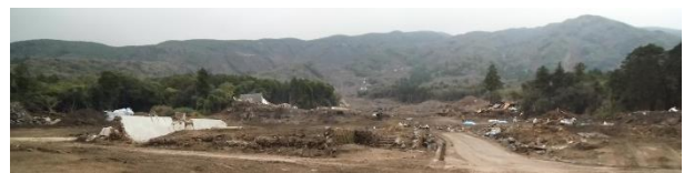
Photo 2 Slope failure and damage (November 9, 2013)
