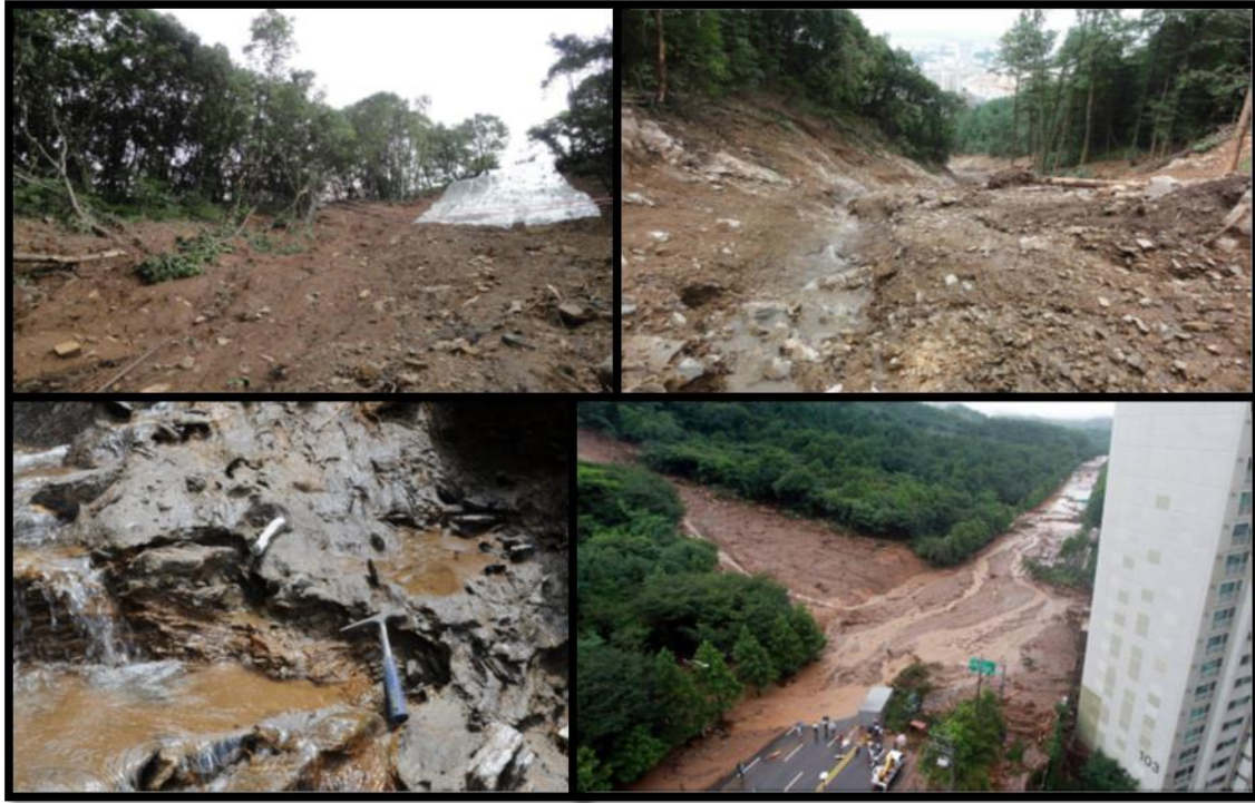
Fig. 2.11. Landslides on Mt. Woomyeon: (A) Landslide scarp; (B) Debris flow gully (entrainment); (C) Ground water table underlying the removed colluvium; (D) Deposition zone (Korean Geotechnical Society, 2011).
