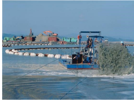
Placement of sheet & hydraulic placement of sand mat
