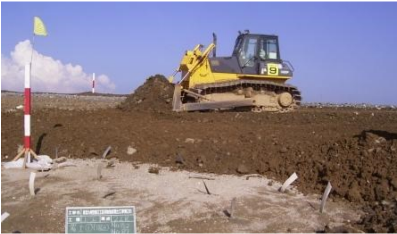
Filling by hill-cut material
