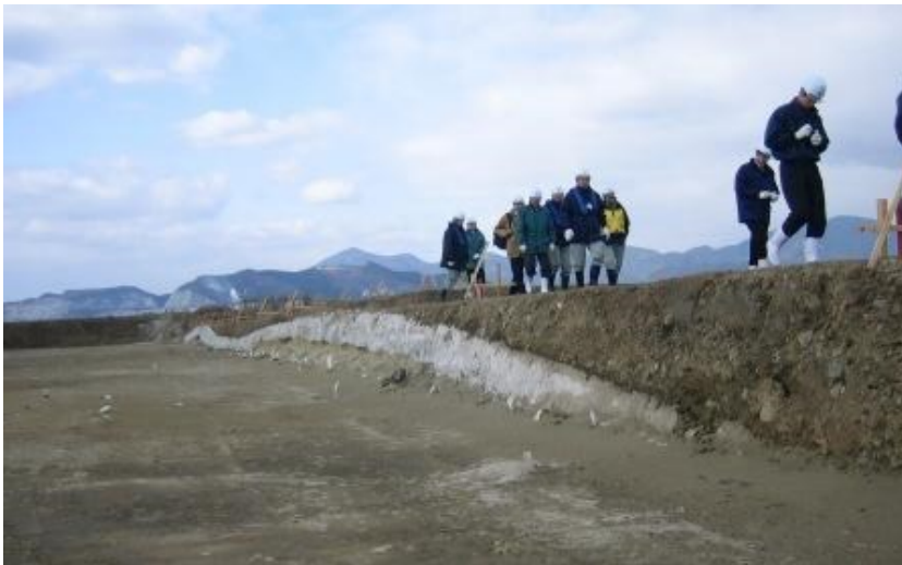
Uneven settlement of reclaimed soil
