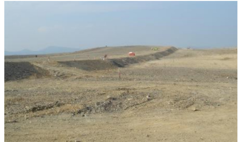
Consolidation of reclaimed clay under the fill
