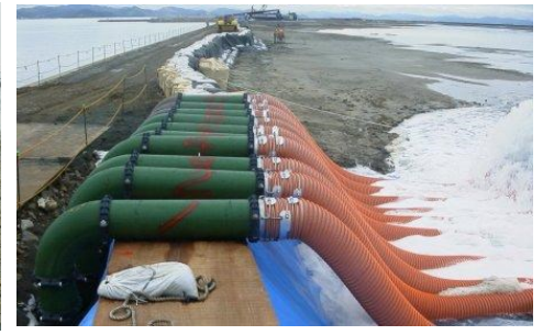
Pouring water for sand mat placement
