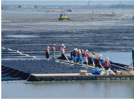
Placement of sheet & hydraulic placement of sand mat
