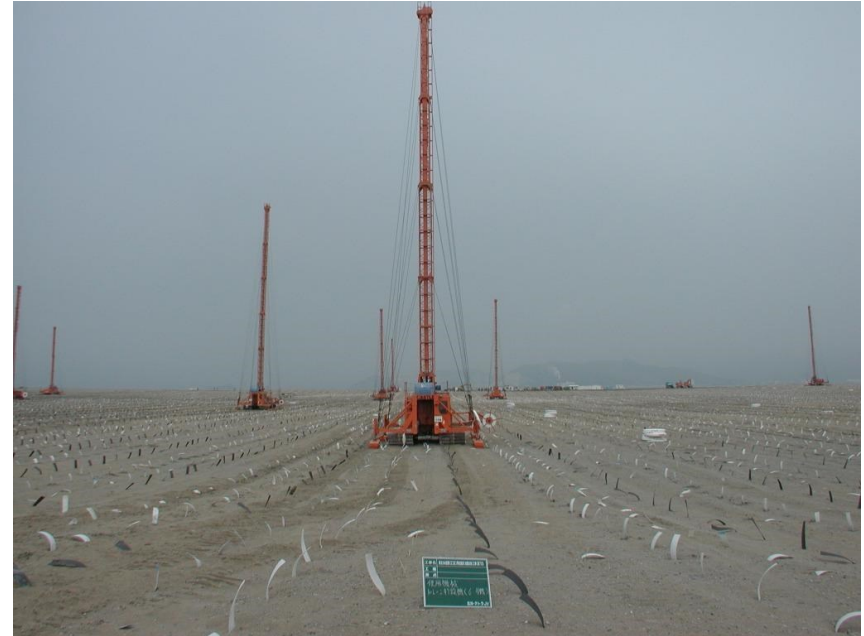
Placement of sheet & hydraulic placement of sand mat
