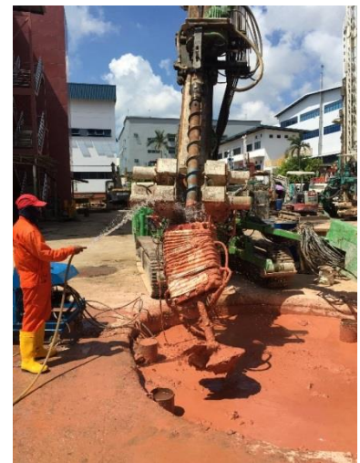
Fig. 3. Field test on an equipment for deep mixing around corners and obstacles
