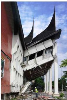
Building collapse, 2009 Padang Earthquake, Indonesia (EEFIT, 2009)
