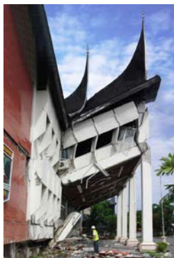
Building collapse, 2009 Padang Earthquake, Indonesia (EEFIT, 2009)
