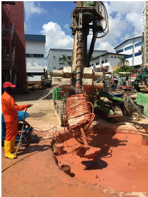
Fig. 3. Field test on an equipment for deep mixing around corners and obstacles.
