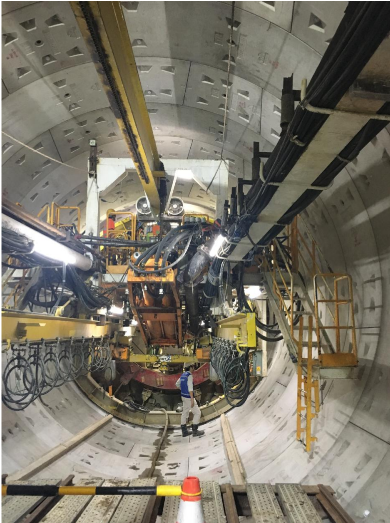
TBM tunneling
