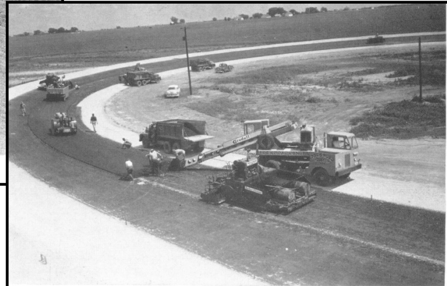
Figure 29. Bituminous concrete construction.
