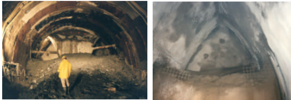
Figure 13: Photographs showing the Himmelberg North Tunnel during excavation: (a) view of the full cross section with side drifts; (b) left side drift (photographs provided by Balbi, 1999)
