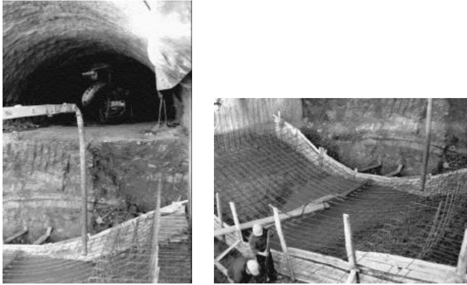
Figure 14: Top heading and benching down excavation method, with placement of heavily steel reinforced invert arch at a short distance from the top heading working face. S. Ambrogio tunnel along the Palermo-Messina Highway in Italy
