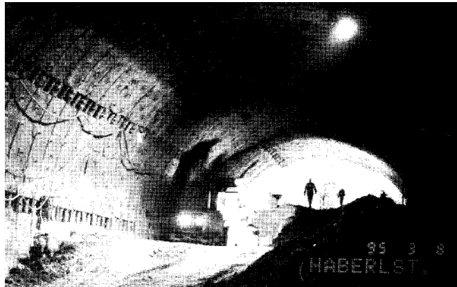
Figure 22: “Galgenberg Tunnel” (Austria), yielding-steel-elements installed in deformation slots of the shotcrete lining (Moritz, 1999)
