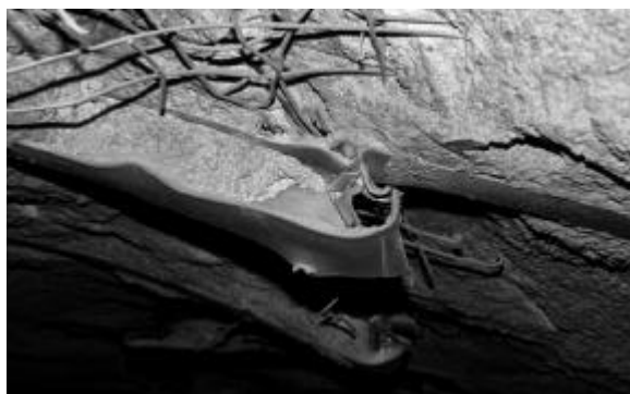
Figure 27: Sheared lining in the Inntal tunnel (Schubert, 2000)
