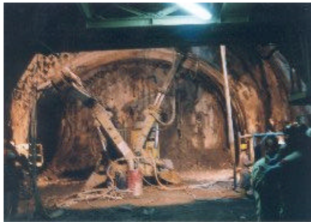
Figure 18: Full face excavation method, Marinasco tunnel near La Spezia, in Italy. Large equipment being used at the face
