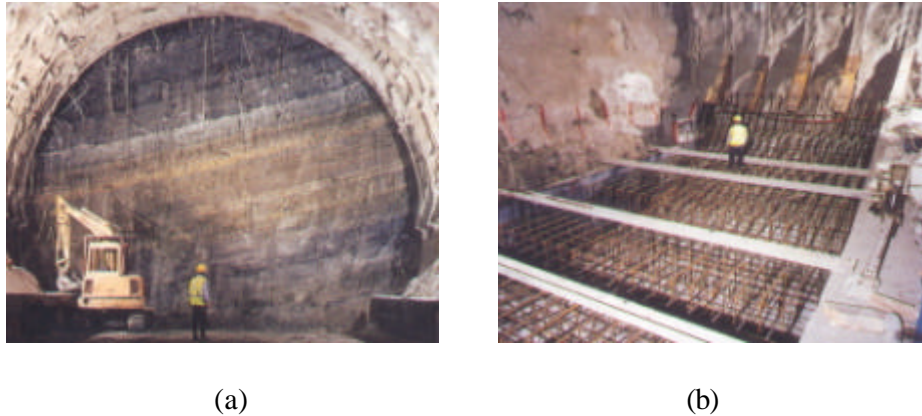
Figure 17: Full face excavation method, Tartaguille tunnel, in France: (a) photograph of the face; (b) photograph of reinforced concrete invert (Lunardi et al., 2000)
