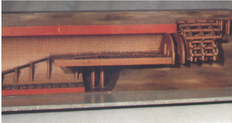
Figure 8: Photograph of a wooden model representing the Belgian excavation sequence in tunnelling (Courtesy of the Politecnico di Torino Museum)
