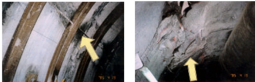
Figure 26: Damaged tunnel lining in the Pinglin pilot tunnel
