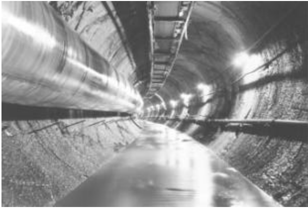
Figure 11. A view of the F2 tunnel in the section where the gneiss rock mass was generally good.
