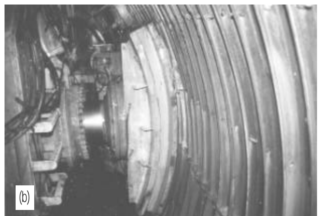
Figure 12. A view of the F2 tunnel: (a) left (b) right walls, where stability conditions became very difficult so as to require continuous placement of liner plates.
