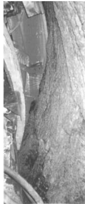
Figure 14. Photograph showing the head of TBM jammed with rock overstressing and block movement of the right sidewall.
