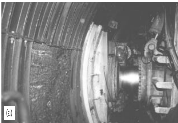
Figure 12. A view of the F2 tunnel: (a) left (b) right walls, where stability conditions became very difficult so as to require continuous placement of liner plates.
