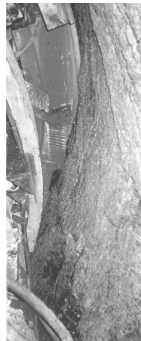
Figure 3. Photograph showing the head of TBM jammed with rock overstressing and block movement of the right sidewall.
