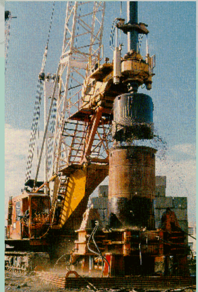
Bored piling rig with bucket auger
