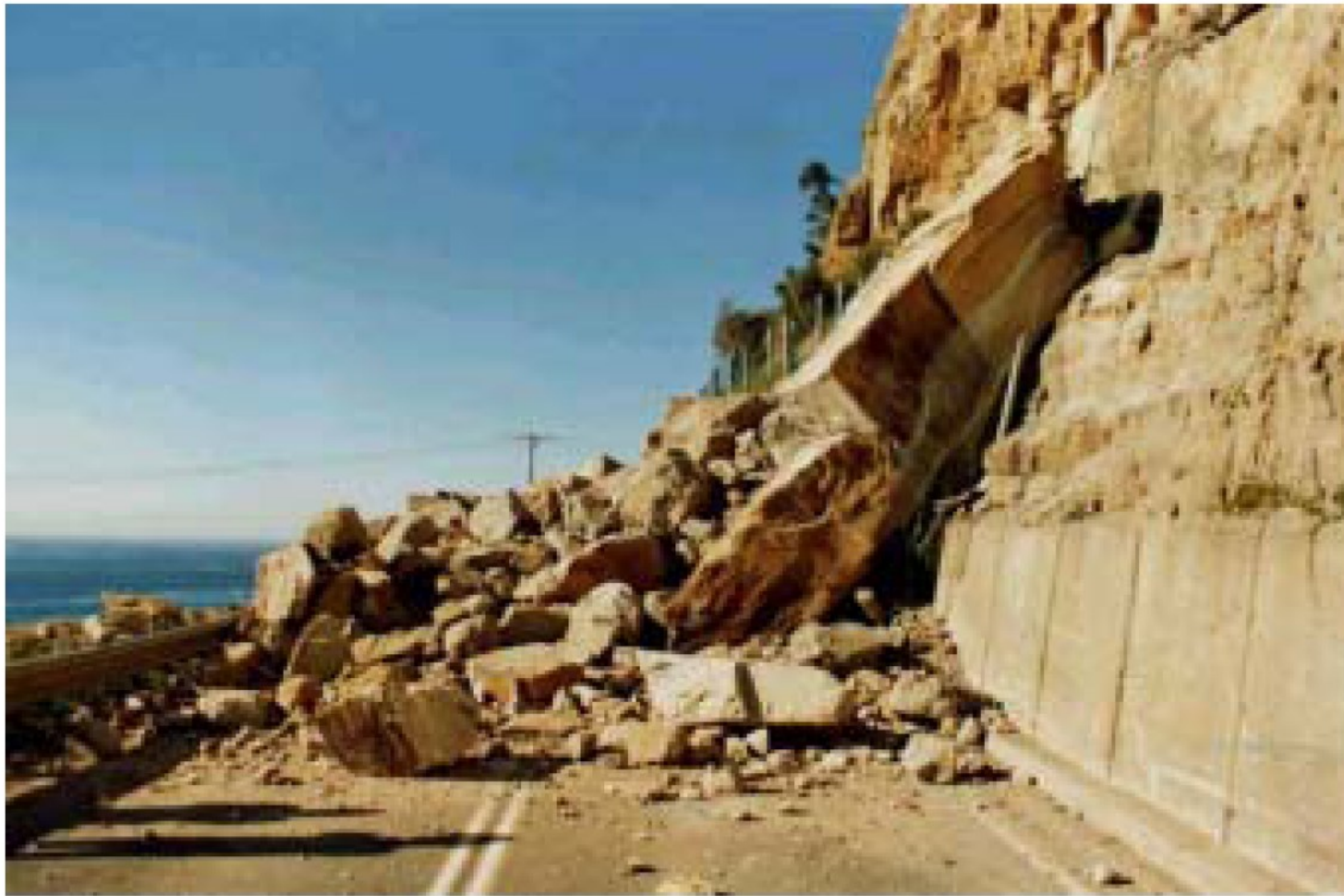
Figure 6. Toe failure below a large slab of Scarborough Sandstone from cliffs in GD1 in 1987 about 90 t of rock.
