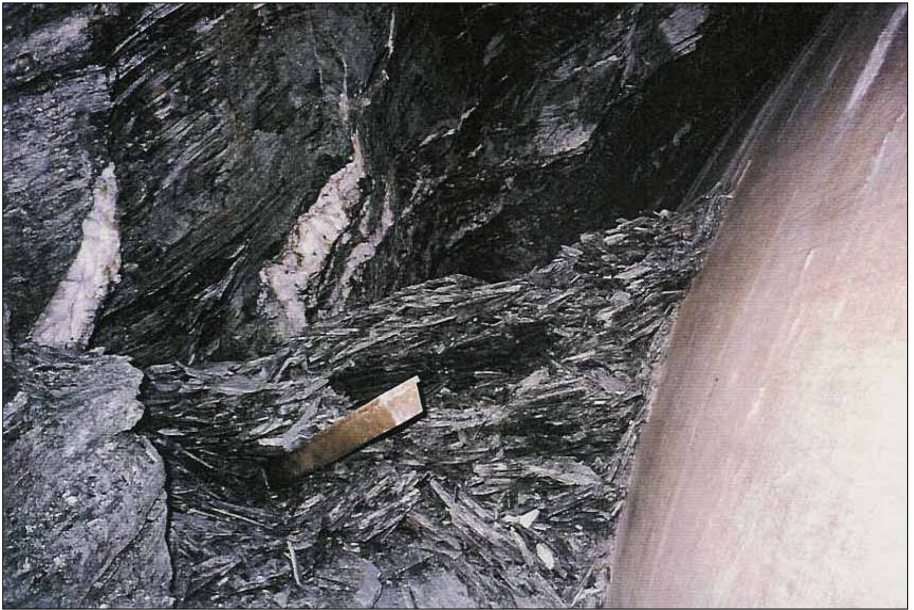
TBM BLOCKED IN THE PHYLLITE.....OVER-EXCAVATION DUE TO SHORT STAND-UP TIME
