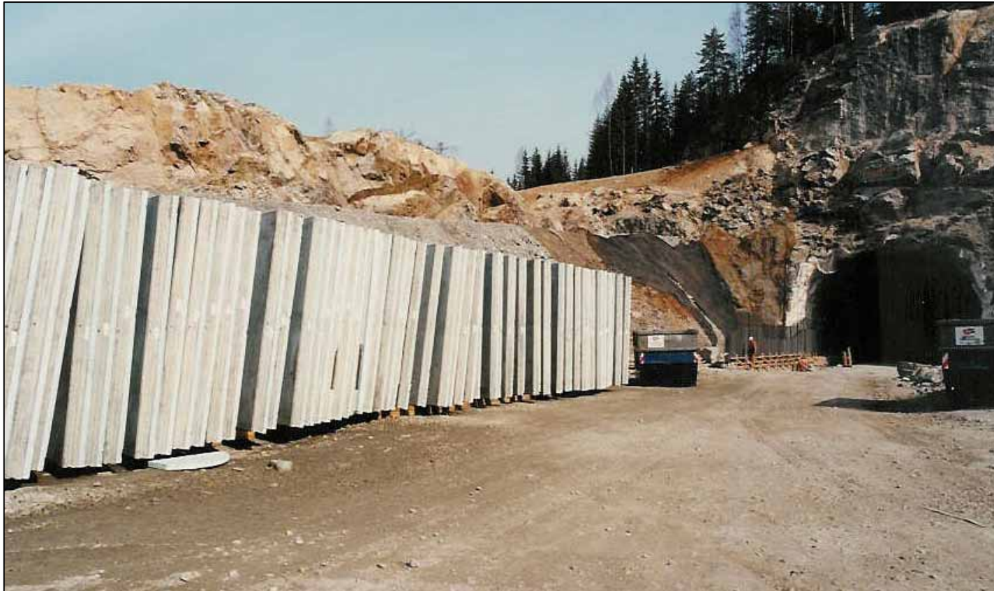
PC-elements stacked at rail tunnel portal ready for mounting with outer membrane sheet – at rates of 900m/month (after learning curve)
