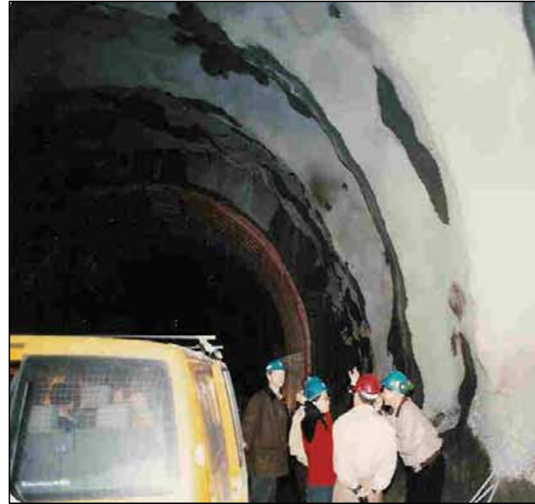
Appearance of ('bent') RRS in subway station location where central pillar was excavated after side-cuts, and in road tunnel ( CCA in background).
