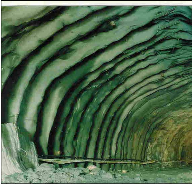
Appearance of ('bent') RRS in subway station location where central pillar was excavated after side-cuts, and in road tunnel ( CCA in background).
